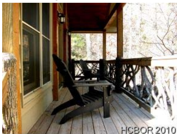
Covered Deck Off Master Suite
